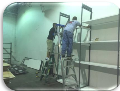
building in progress...
